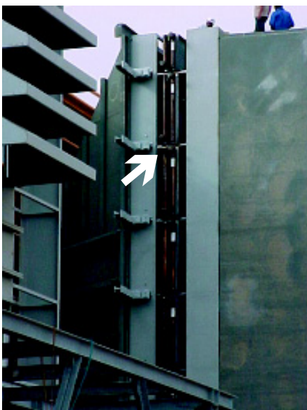
The Donaldson Chiller Coil System typically occupies a space between the filter house and the transition.
