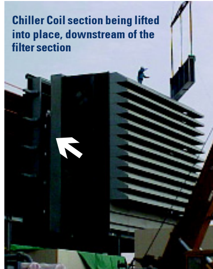
The Donaldson chiller coil system being installed will cool the inlet air for a GE Frame 7EA Gas Turbine in the hot, dry desert environment near Onaizah, Saudi Arabia.
