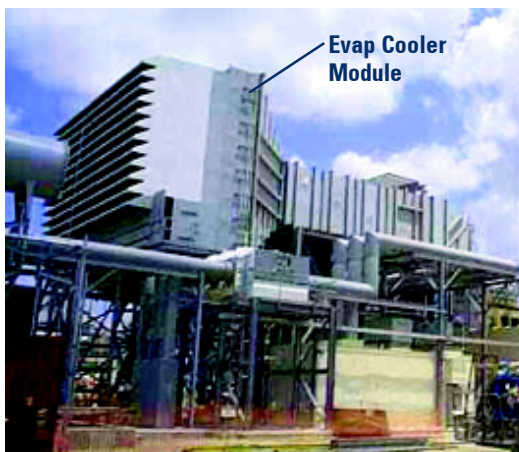
Donaldson's Evaporative Cooler fits neatly behind any of the Donaldson air inlet filters -- in this case it's downstream of a GDX self-cleaning filter.
