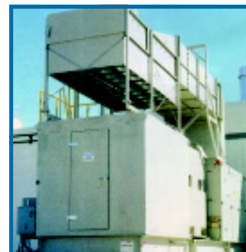
TTD self-cleaning air filter protects a Solar turbine in the hot, arid, dusty environment in Nevada USA.
