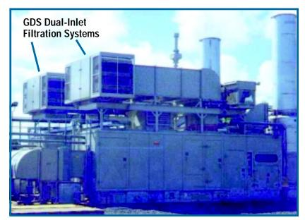
These Donaldson Dual-Inlet GDS Filter Systems protect turbines from the ravages of sand and dust near Tucson, Arizona USA. Note the insect screens over the inlet hoods. Donaldsn GDS systems keep combustion air clean for hundreds of turbines all over the world.
